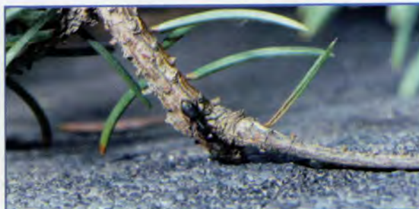
Figure 5. Branches overhanging and touching homes can provide carpenter ants access to houses.
