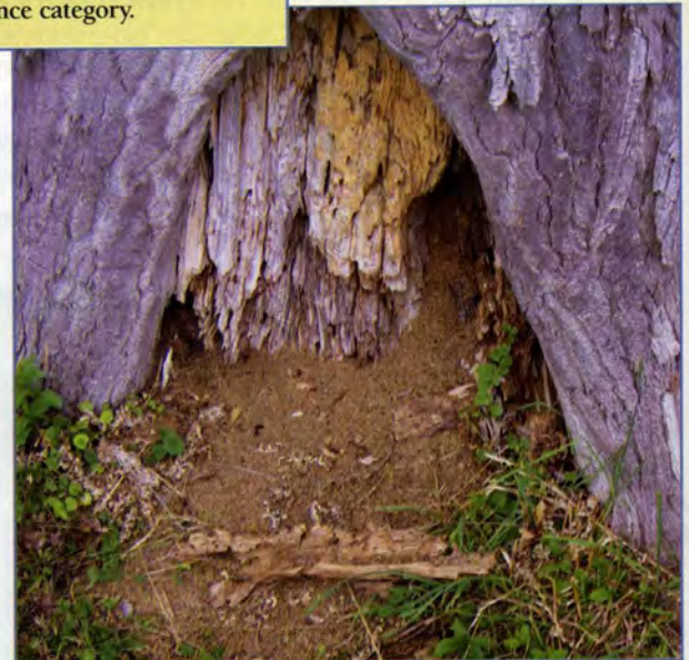
Figure 2. The presence of carpenter ants in living trees is an indicator of the presence of decay.
