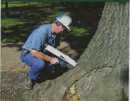
An oak tree is tested for decay with a Resistograph.
