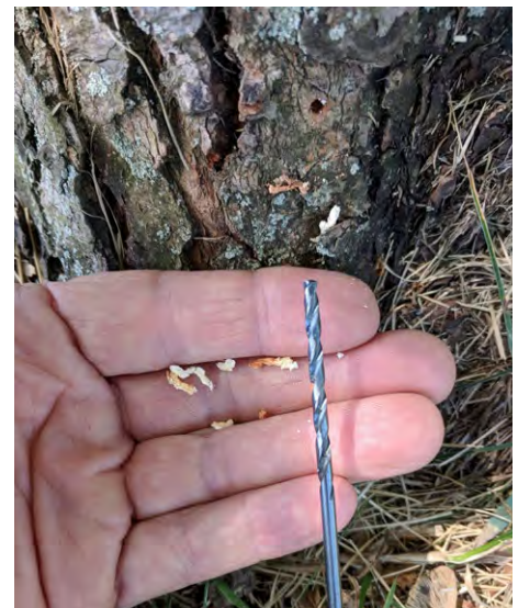
Photograph 5. Drill extraction of decay with a small diameter drill bit provides an adequate sample.
