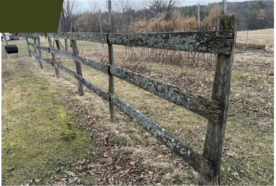
Photo 1: Man has used the increased resistance of heartwood of some tree species for wood in service. Here, black-locust fence posts and white-oak rails have resisted decay in service for more than 20 years. Unless otherwise noted, all photos courtesy of Christopher Luley.
